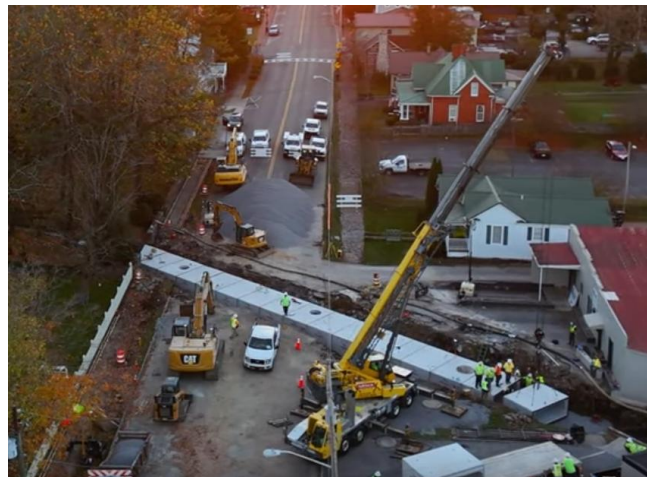
Figure 2. Box Culvert Replacement under East Main Street, 2024
