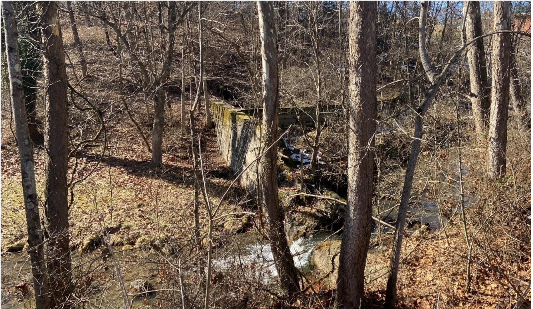
Figure 13. Mill Dam along Wolf Creek
