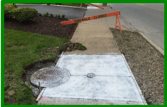
Sidewalk Rehabilitation Program
