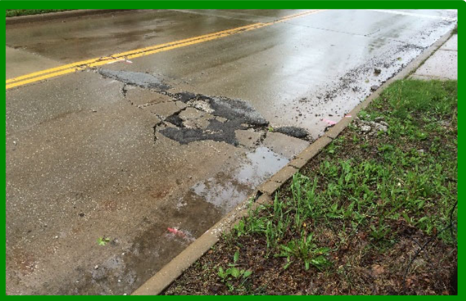
Dover Center Road Resurfacing – Center Ridge Road to North Olmsted Corporate Line
