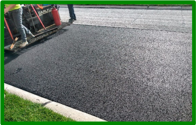
Crocker Road Resurfacing – Detroit Road to Hilliard Boulevard
