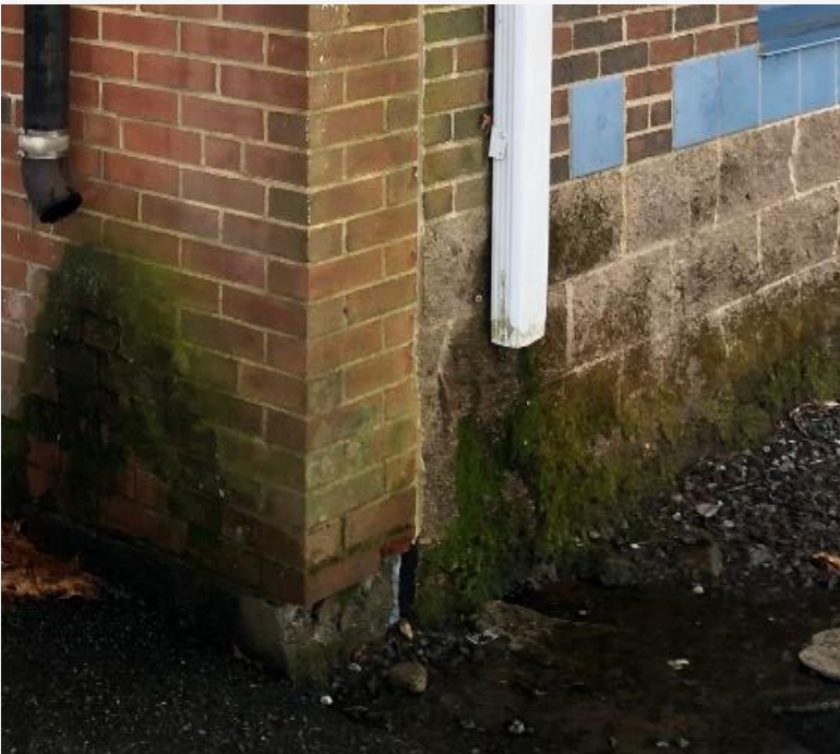
Deteriorating/Cracking Masonry
