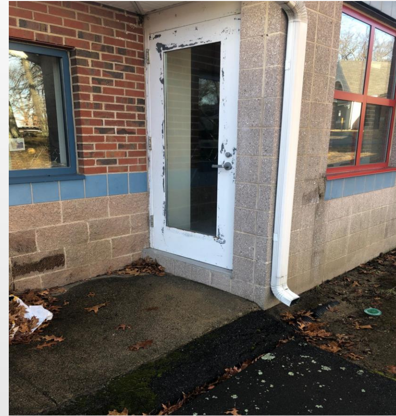
Non-Accessible Exterior Doors
