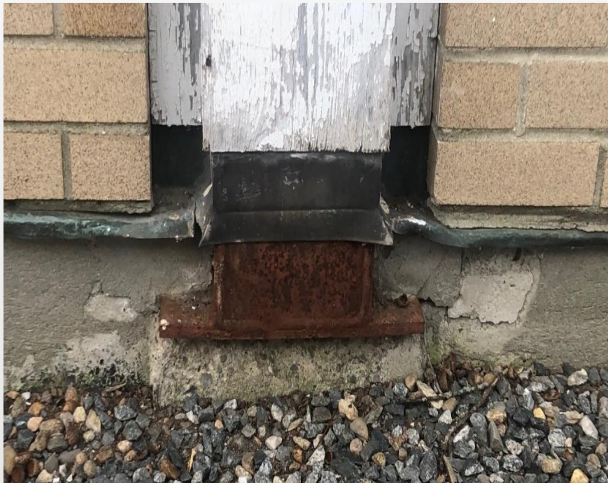
Exposed Steel Columns
