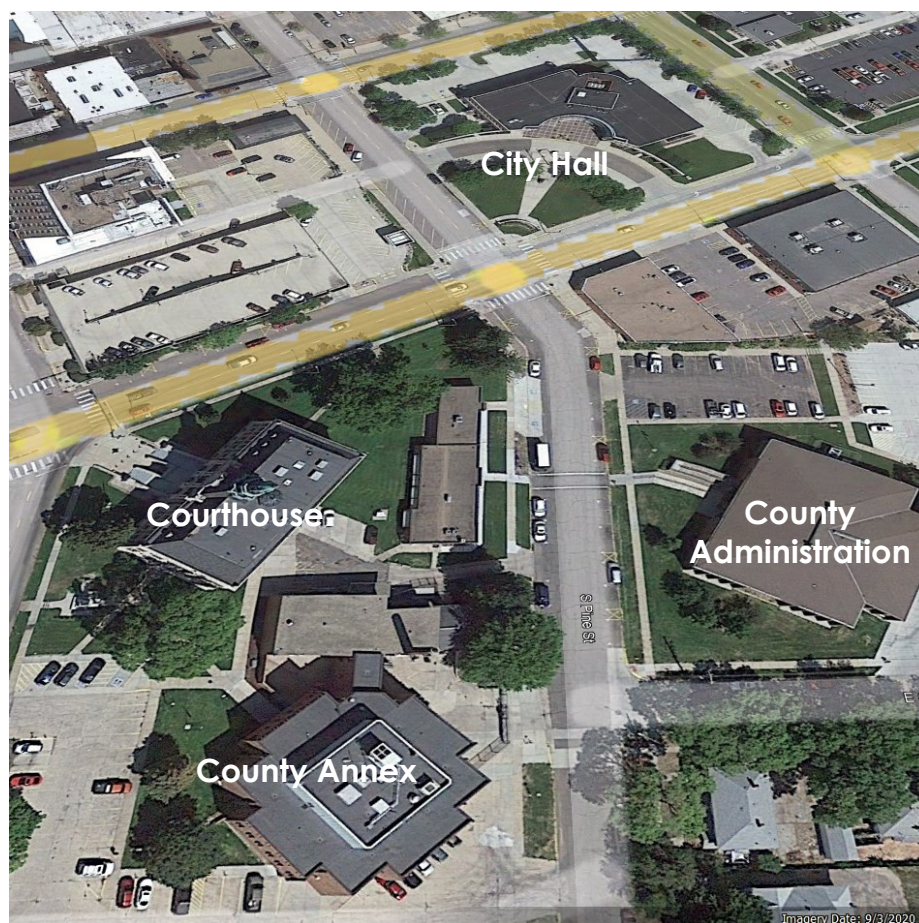
Figure 6.1: Grand Island City Hall and Hall County Courthouse
