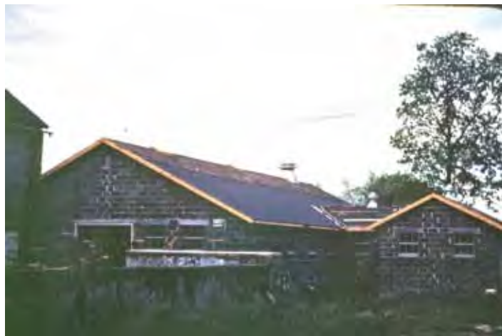
The existing maintenance shed was built in 1949, originally used as a cattle stable.
