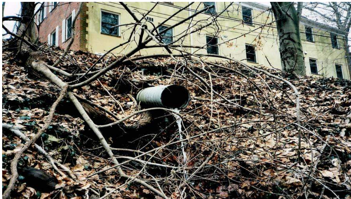
Stormwater outfall pipe, slope of Thorntown Creek floodplain, behind Third Street
