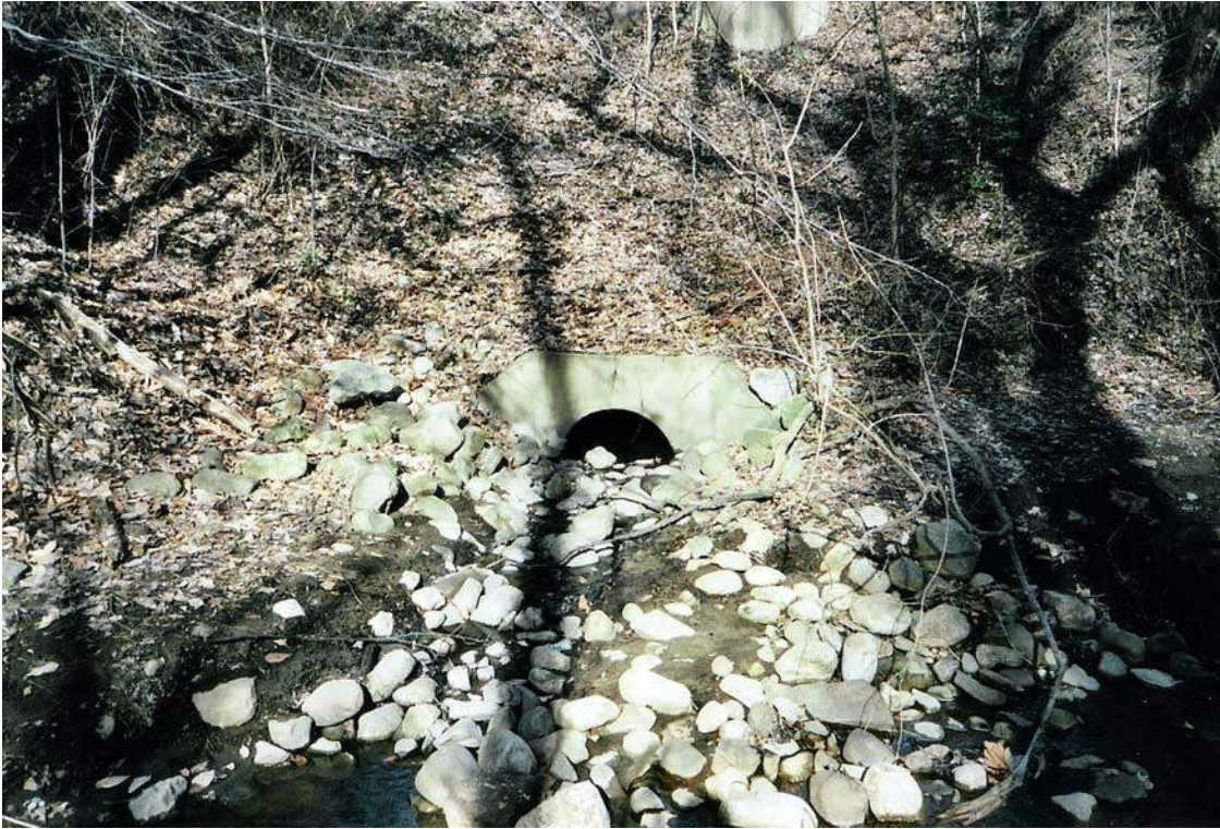
Detention basin outfall (from Ocean Spray property), Thorntown Creek
