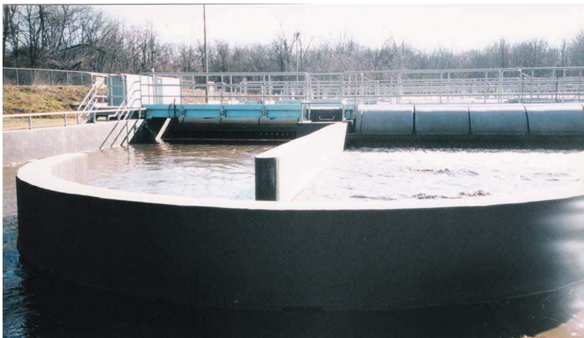
Bordentown Sewerage Authority treatment facility
