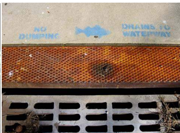
Storm Drain Inlet, East Burlington St. Note
