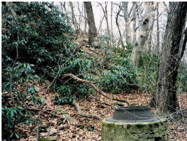
Rhododendrons, Thorntown Creek (abandoned stormwater manhole in foreground)
