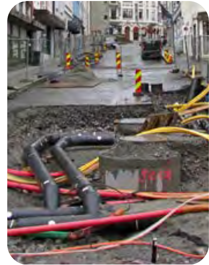
Underground Utilities Construction. Source: 4M Analytics
