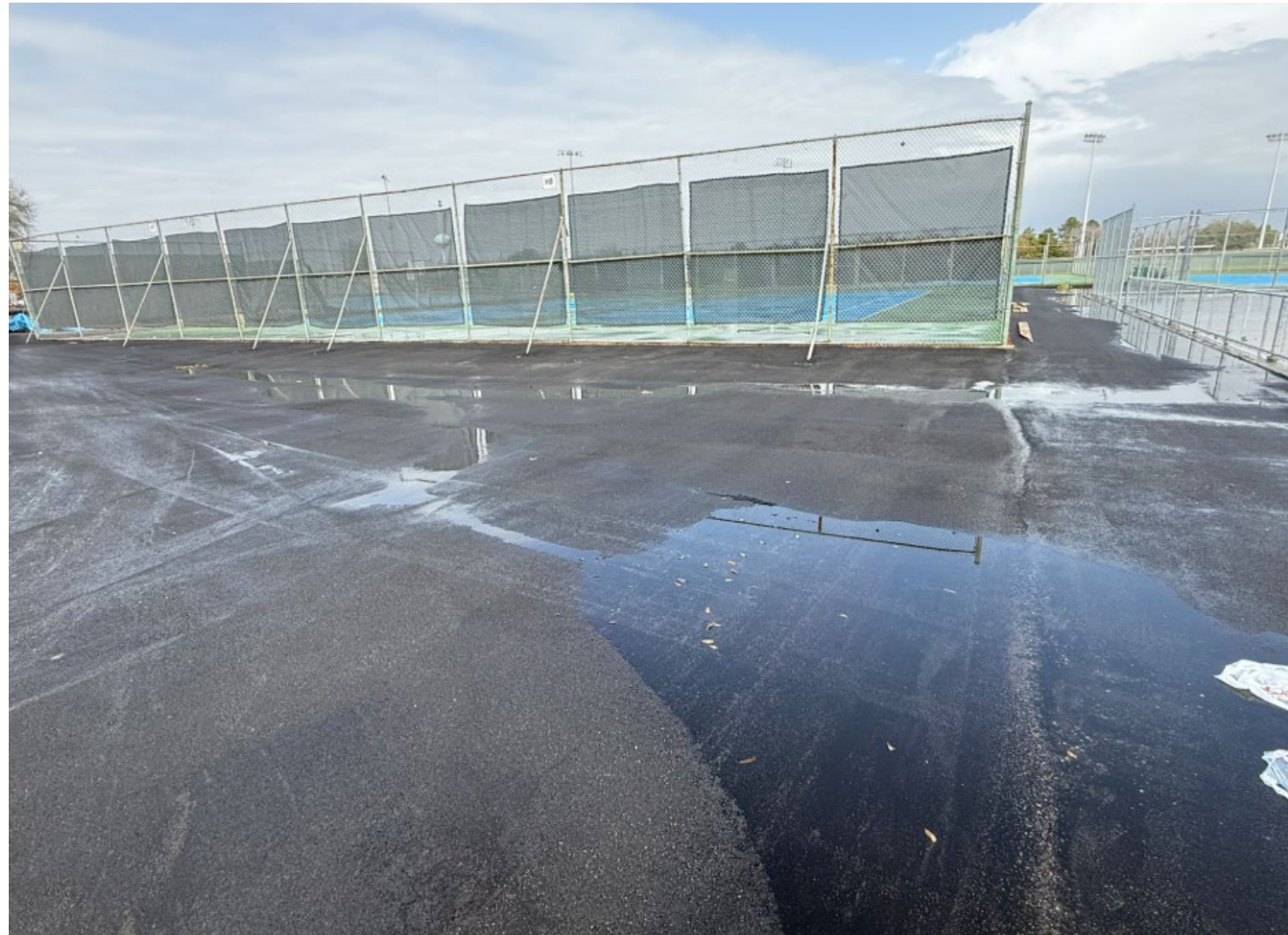
Tennis Court Picture of new asphalt and fencing
