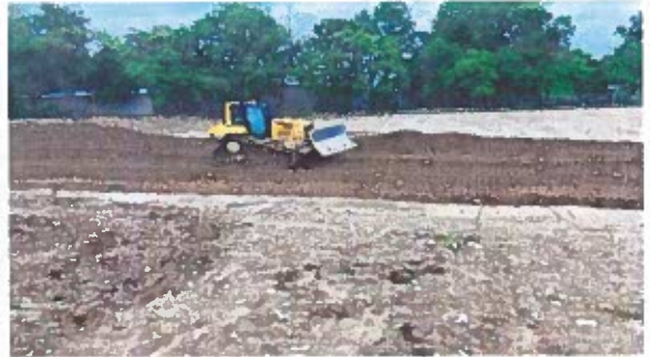
Site grading in progress
