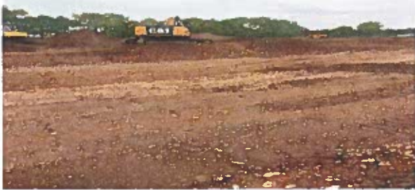
Topsoil being removed from site
