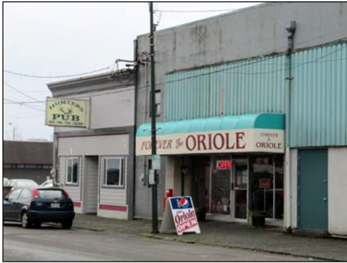
No. 31 The Oriole Café, 708 J Street, occupies part of the former J. C. Penny Building (1928). The former department store, at 411-417 7 th Street and the corner of 7 th and J Streets, also houses the offices of a dentist and an eye doctor to the north of the Oriole Cafe.
