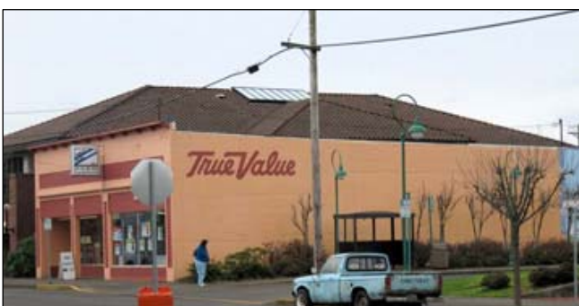
No. 28 The building housing the True Value Ace Hardware, 414 7 th Street, dates from 1912.
