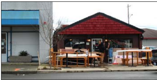
No. 17 The 8 th Street Ale House, at 207 8 th Street, was recently rehabilitated. The narrow deep structure expresses the original platting of parts of its block.
