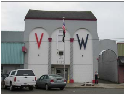
No. 29 The VFW Hall, at 407 7 th Street (1928), is an eclectic style concrete structure with monumental engaged columns supporting an arcade. The building facade has been extended on the west side to encompass and drive entry.
