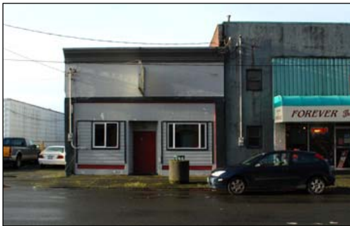
No. 32 The building housing Hunter's Pub, at 710 J Street, reportedly dates from 1908.
