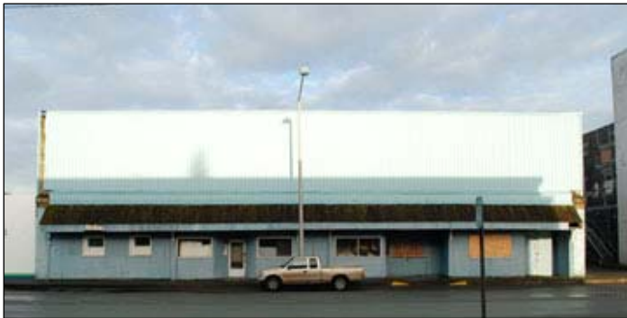
No. 12 The Arnold Block, 516 8 th Street, is a two-story unreinforced brick structure dating from 1911. This building has considerable historic significance due to its association with F. D. Arnold, an early banker and businessman who promoted the city and constructed the building. (See historic photos on page 14.)
