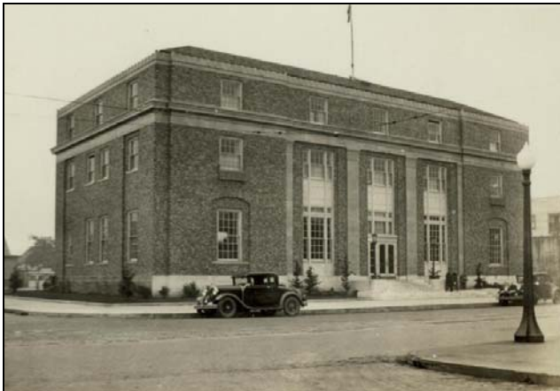
Historic images of important buildings in downtown Hoquiam, left.
