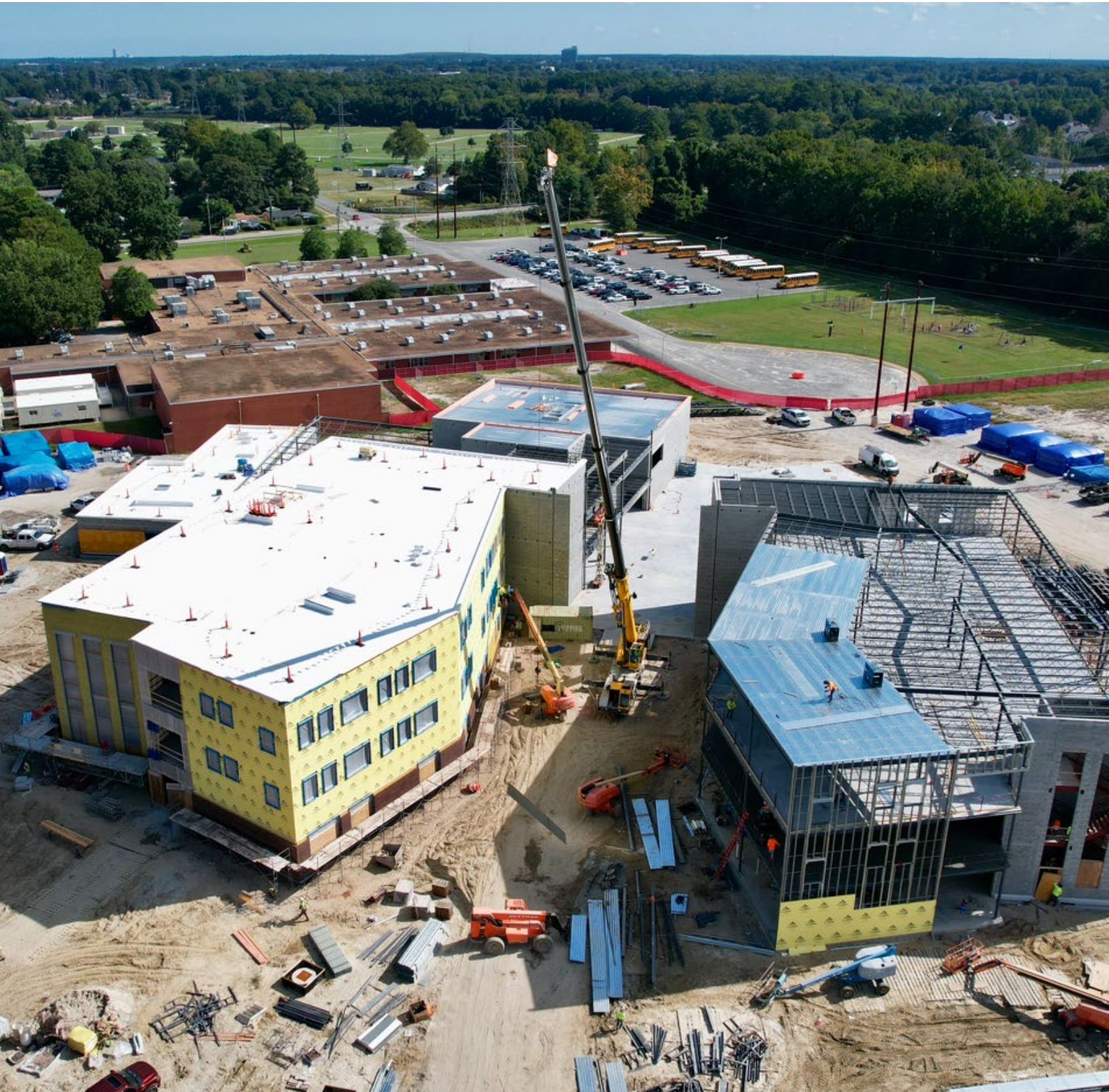
New Crestwood Elementary School
