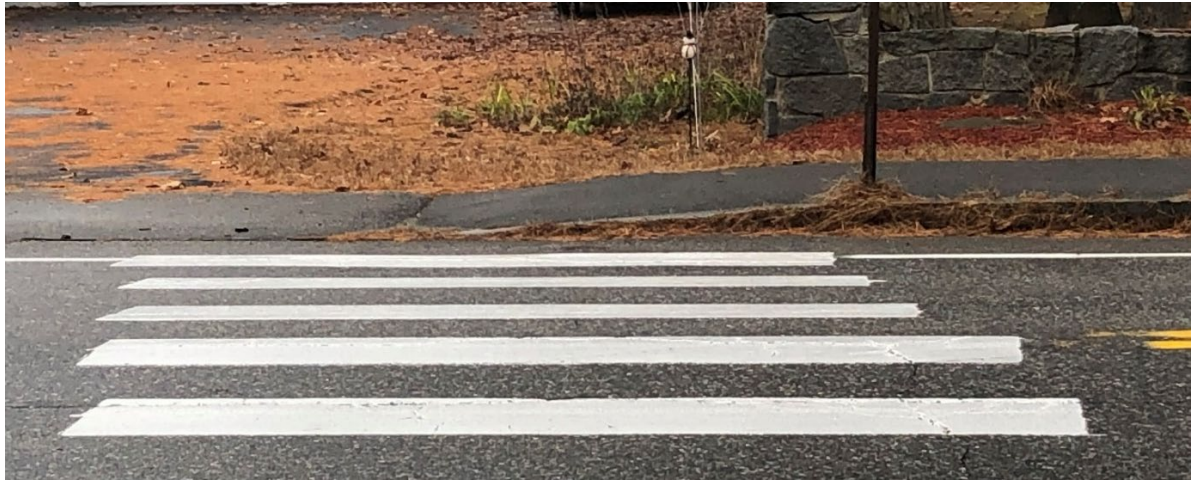
Photo 1: West Side of East Side Drive Crosswalk at Portsmouth Street Intersection
