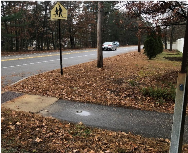
Photo 11: From South Curtisville Road Looking to the North on East Side Drive
