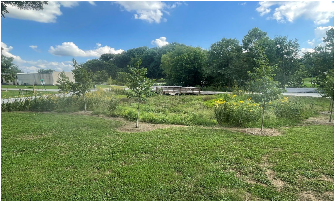
Figure 17. This bioretention area in Siloam Springs was funded through the Riparian Restoration Program and captures, infiltrates, and treats stormwater from 10 acres of impervious surface before draining into Sager Creek.
