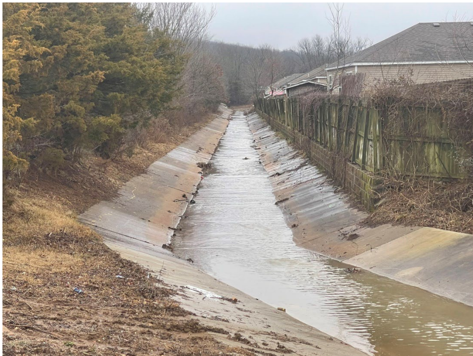
Figure 15. Concrete channel along Spring Creek near Ford Avenue
