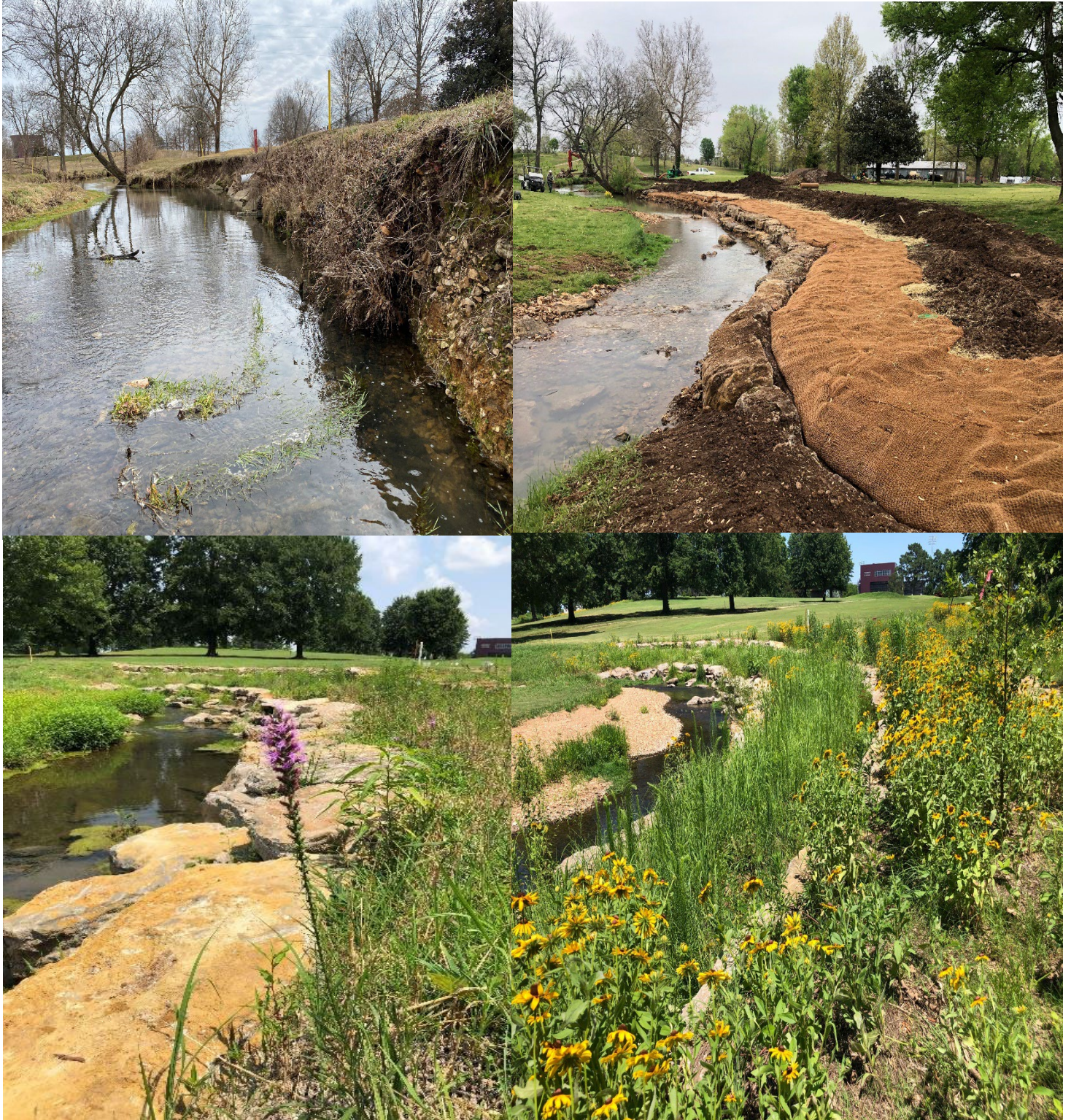
Figure 19. Pictured above are photos of before, during, and after construction of Natural Channel Design streambank stabilization project at the Course at Sager's Crossing, located in Siloam Springs. Soil lifts were also implemented and planted with native vegetation to create additional floodplain connectivity. This project was funded through IRWP's Riparian Restoration Program in 2021.
