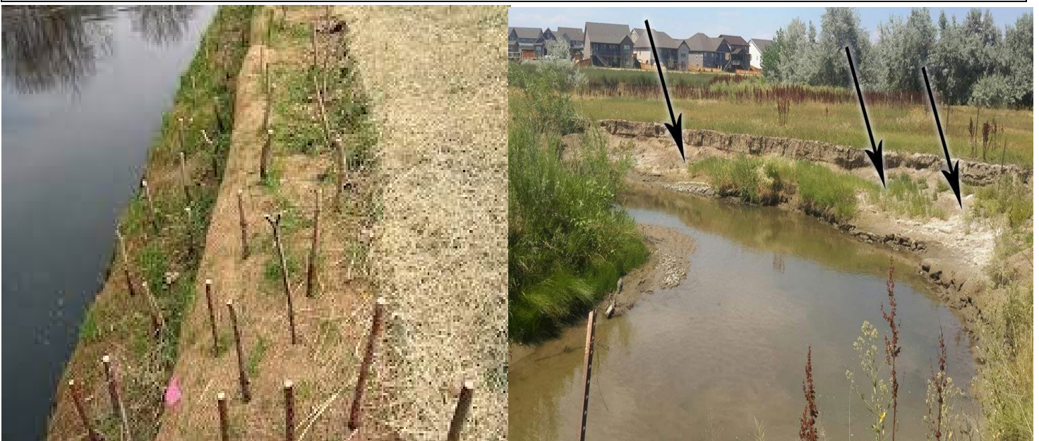
Figure 4. Moderate streambank erosion along the spring fed tributary of Spring Creek (pictured above), north and south of Fleming Drive bridge. Implementing native live stake cuttings (pictured below) as well as a mix of conservation grade trees, shrubs, and herbaceous perennials adapted to local Riparian Zones 1 and 2 would armor these streambanks in 1-2 years, protecting them from future erosion and creating important aquatic and terrestrial wildlife habitat.
