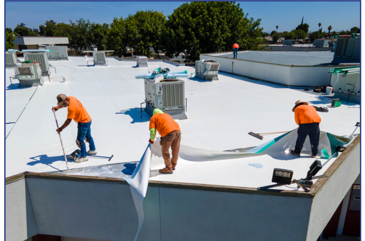
Above, workers reroof the 600 classroom wing at Mae Hensley Junior High – the first in a lineup of projects funded through Measure Y. At left, a classroom wing takes shape at Sam Vaughn Elementary.
