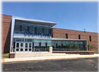
Courtland HS Renovation
