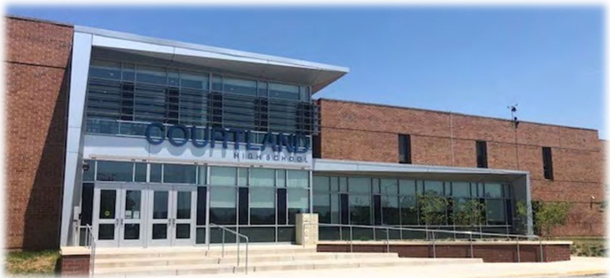
Courtland High School Renovation
