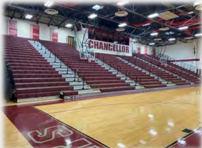
Athletic Facility Improvements
