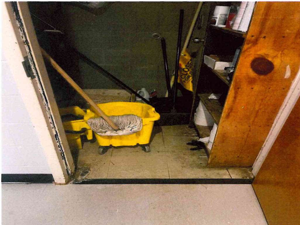
Floor Tile(12x12)w/Mastic: Janitor Closet 4 th Floor
