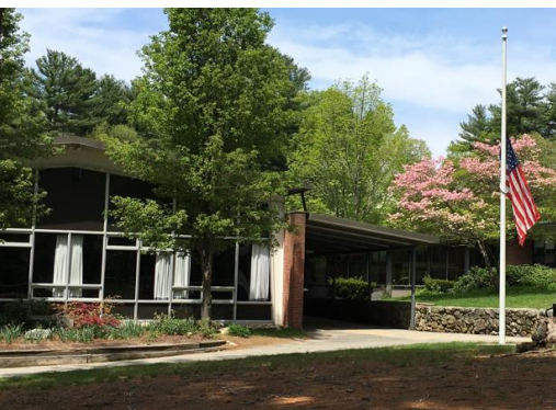
South Elementary School: 1958/1965
