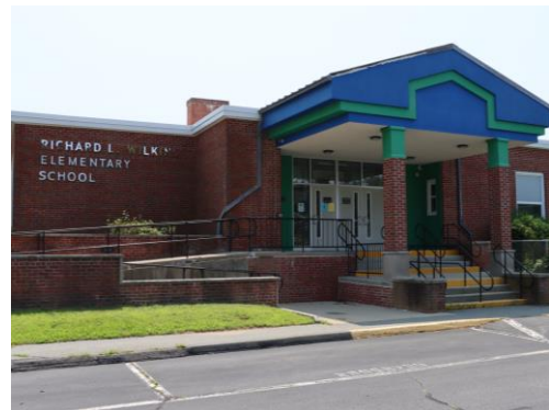
Wilkins Elementary School: 1954/1962
