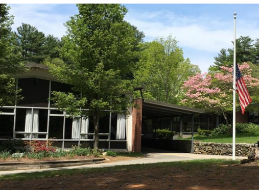
South Elementary School: 1958/1965
