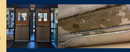
During rain storms, the library entrance leaks from the roof and automatic doors down into the staff kitchen below. These leaks have consistently caused water damage to the ceiling tiles and created safety concerns with wet floors and counters. Warrant Article 25 will allow us to repair these leaks to prevent further damage.
