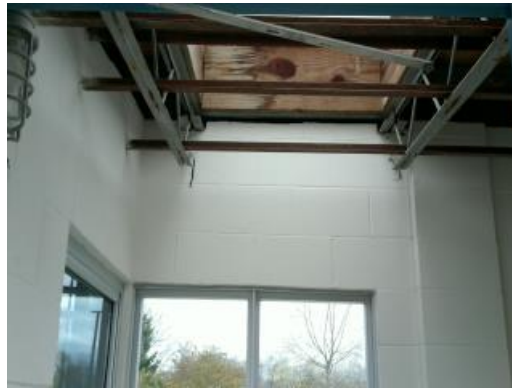
Ticket Booth Exposed Deck Ceiling
