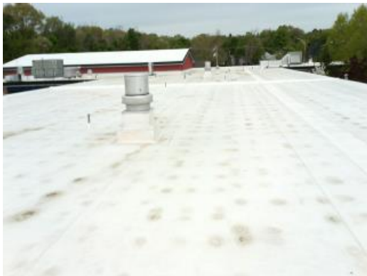
Typical Roof Condition
