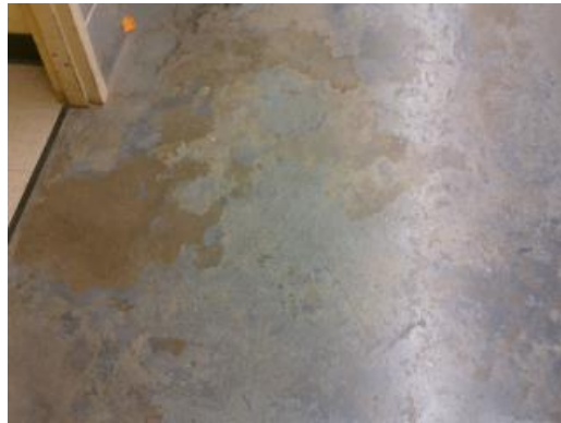
Refinish Concrete Flooring
