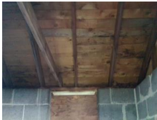
Shed Exposed Wood Ceiling
