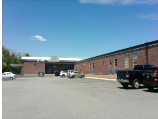
Back of Kitchen
