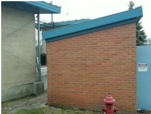
Utility Building-2 Side View
