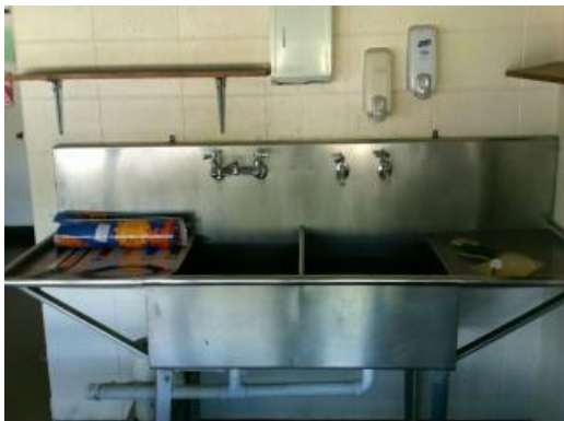
Sink in Room 164
