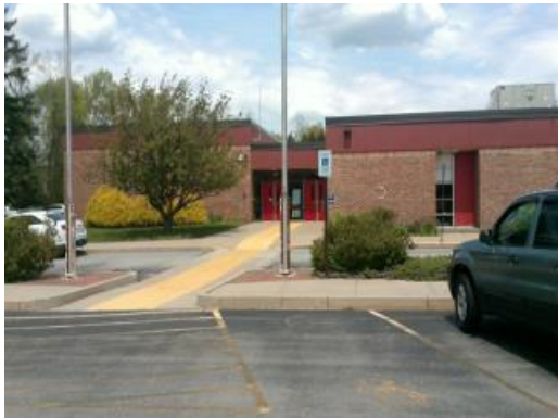
Front Of Building
