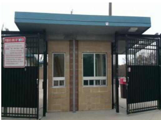
Ticket Booth Front View
