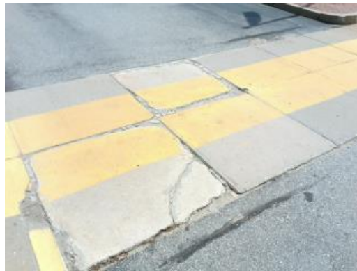
Concrete Walkway At Entrance
