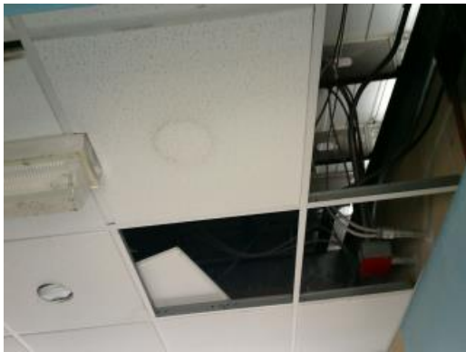
Press Box Acoustical Tile Ceiling
