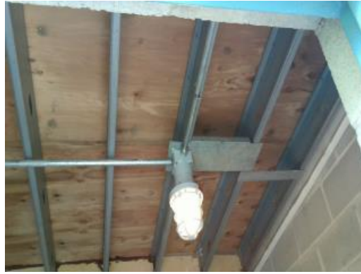
Utility Building Deck Ceiling
