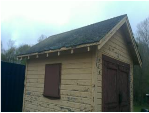
Storage Shed Shingle Roof
