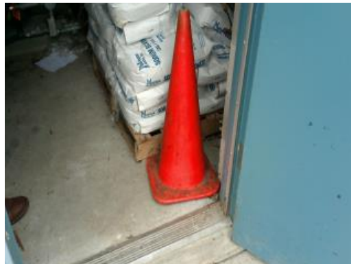
Utility Building Concrete Flooring
