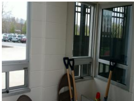
Ticket Booth Interior
