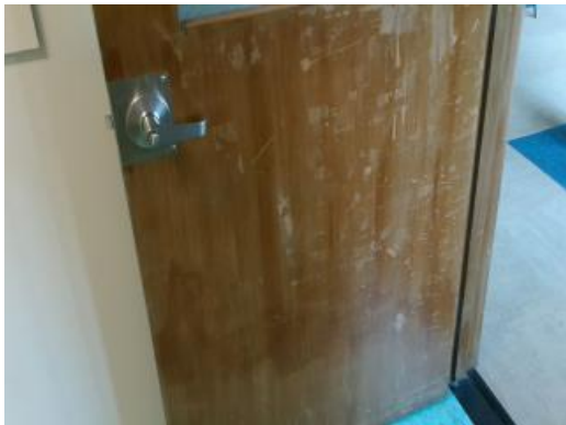
Interior Wood Door
