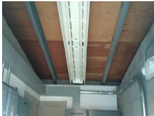
Utility Building-2 Wood Deck Ceiling
