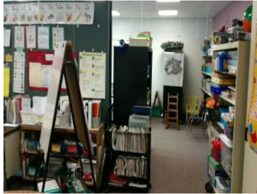
Damaged Carpet At Classroom 22
