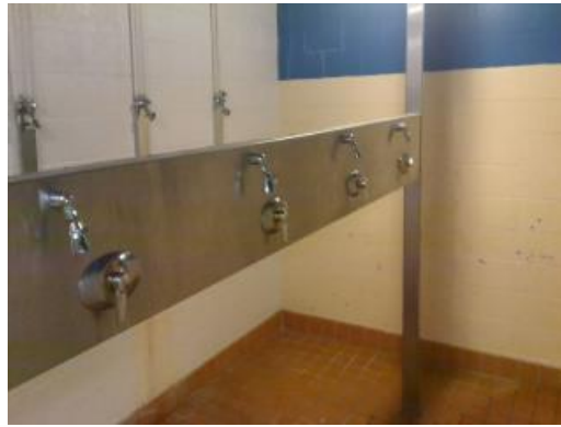
Typical Shower Room
