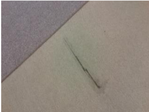
Worn And Tearing Carpet
