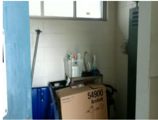
Restroom Utility Room
