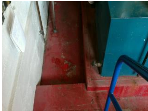
Boiler Room Floor
