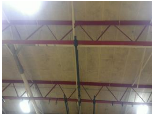
Stained Tectum Ceiling in Gymnasium
