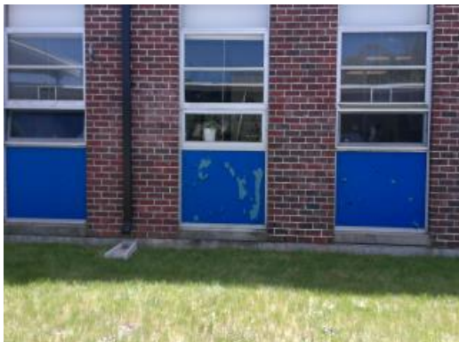
Typical Exterior Windows
