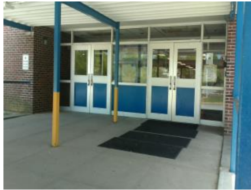
Aging Exterior Storefront Doors
