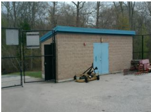
Storage Building Exterior
