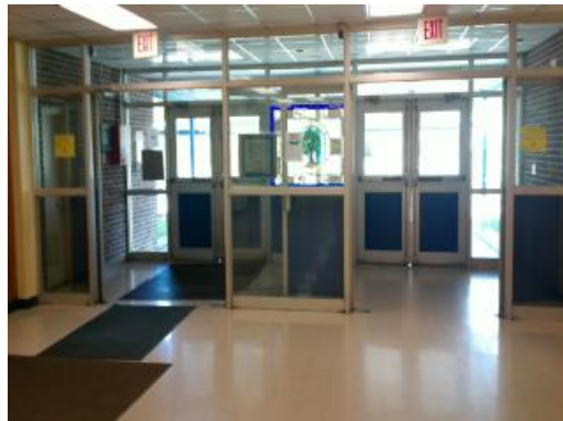
Original Storefront Doors at Front Lobby
