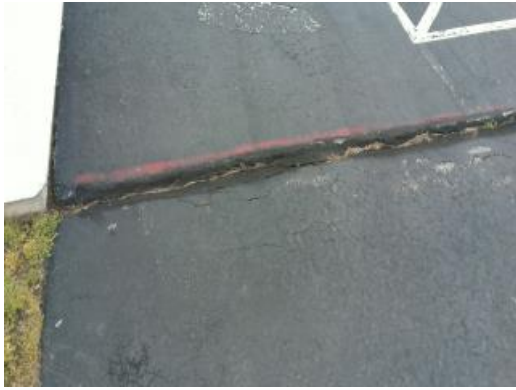
Splitting Asphalt Play Area
